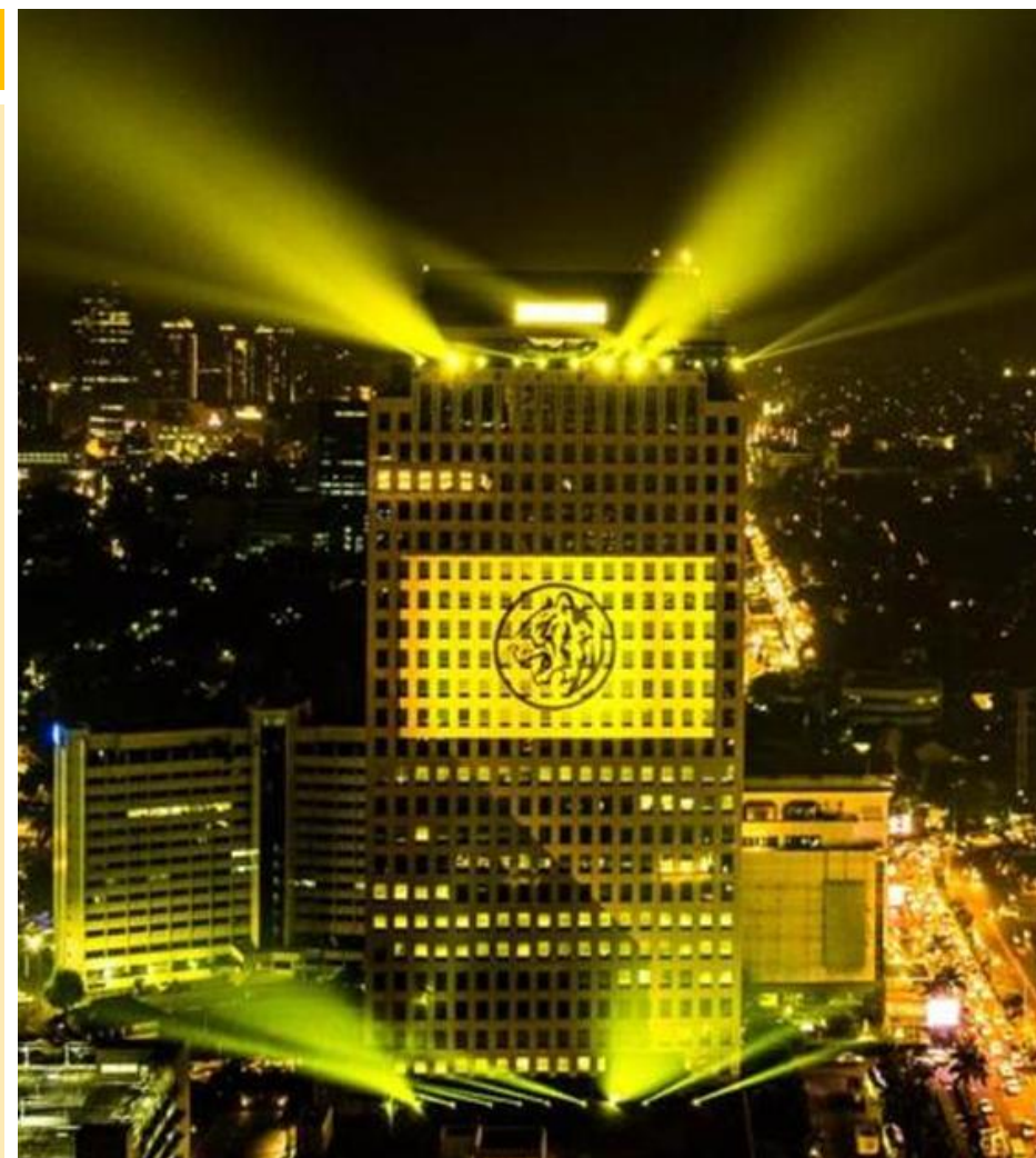
Maybank Indonesia Head Office, Sentral Senayan 3, Jakarta, Indonesia
