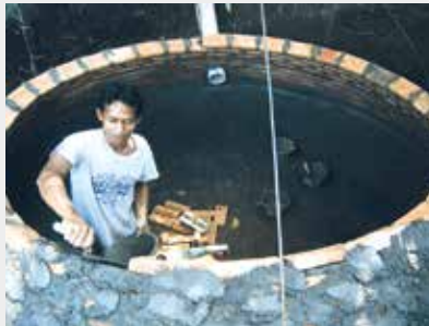
Program Biogas Program Biogas
