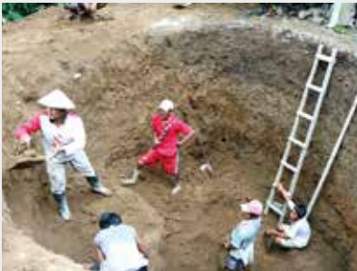
Program Biogas Program Biogas
